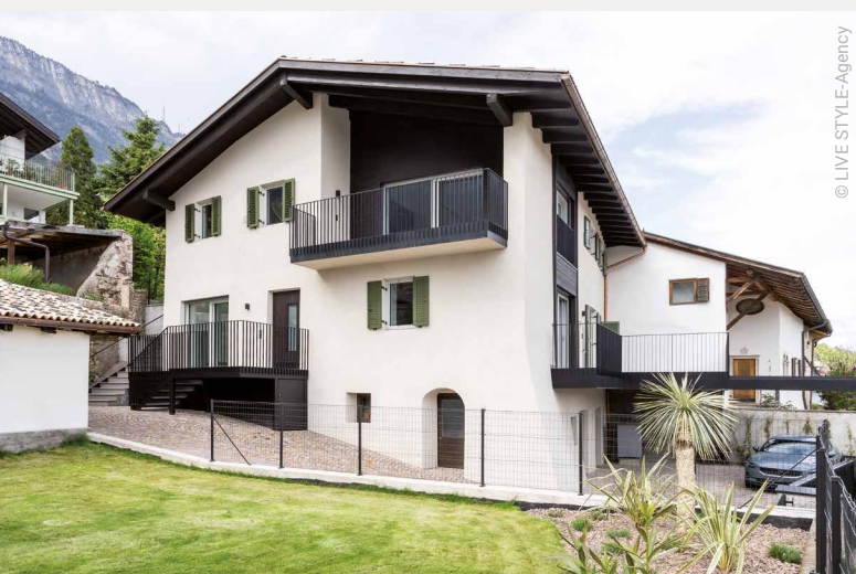
Haus SR | Casa SR Kaltern (BZ) / Caldaro (BZ)
